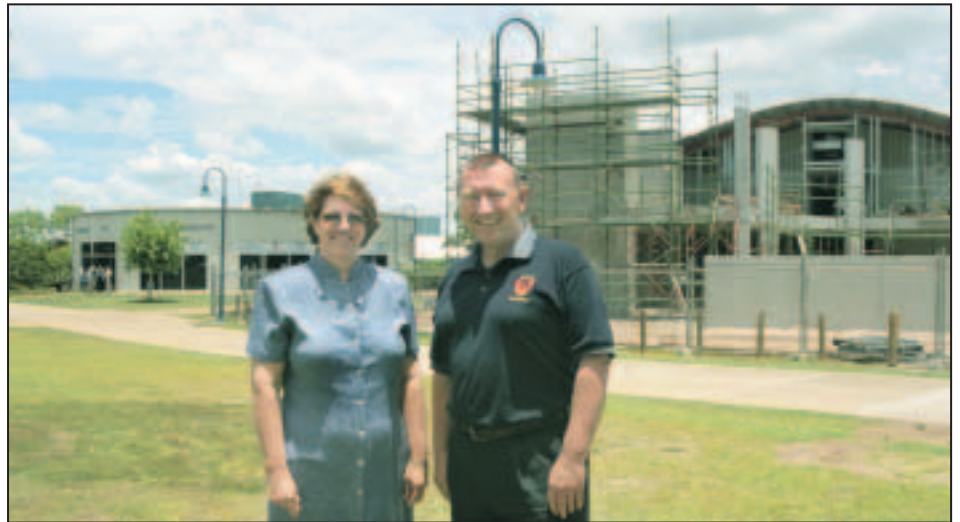
BAY EXPANSION: Construction continues on Stage Two of the development at USQ's Wide Bay Campus. The new Sciences Building will be ready for occupation by the start of Semester One, 2003. In the campus precinct taking a particular interest in the construction are USQ Wide Bay Nursing Coordinator Dr Trudy Yuginovich and USQ Wide Bay Executive Officer Peter Carey. The new building will house laboratories, lecture rooms, and offices as well as nursing practice areas on the ground level of the complex.
