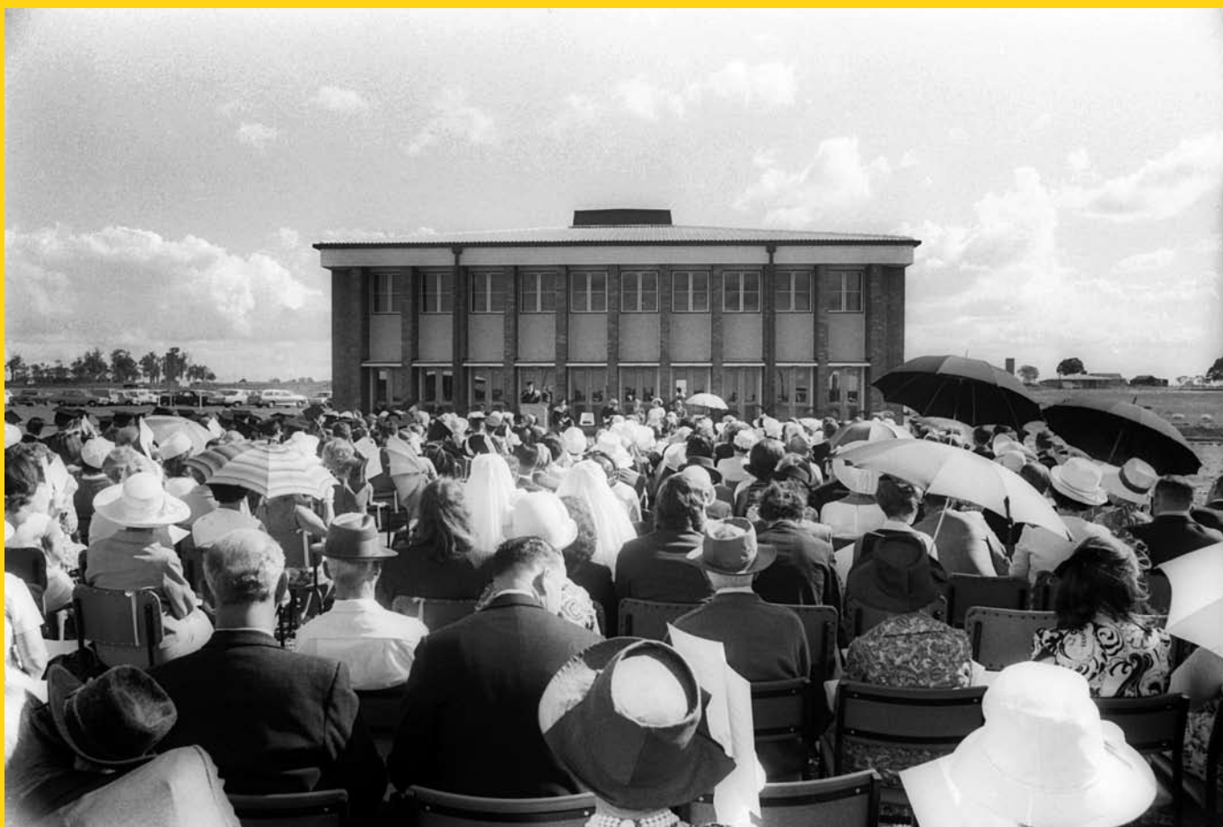
A roof for our students' heads The official opening of the McGregor College in 1971.
