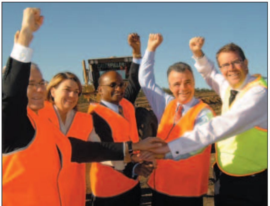
PUNCHING THROUGH: Dignitaries at the groundbreaking ceremony for USQ's Springfield campus celebrate the beginning of construction work at the site. They are (from left) Vice-Chancellor Professor Bill Lovegrove, Queensland Minister for Education and the Arts, Anna Bligh, Maha Sinnathamby (Chairman, Springfield Land Corporation), Federal Minister for Education, Science & Training, Dr Brendon Nelson, and Nick Collishaw (Executive Director, James Fielding Group).
