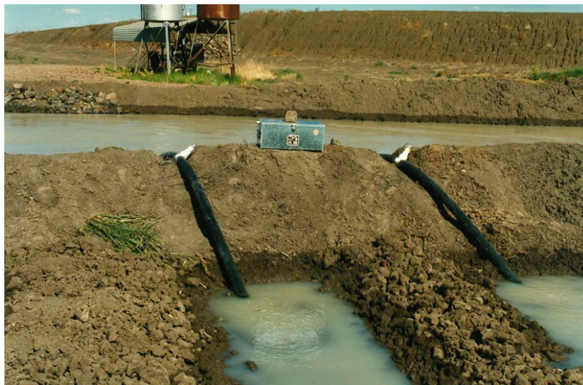
Figure 7: GLI tee-mount meter in irrigation siphons measuring water applied
