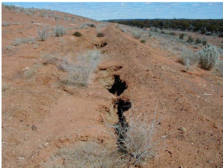
Figure 1. Tunnel developed from a berm on a waste rock dump constructed of sodic spoil.
