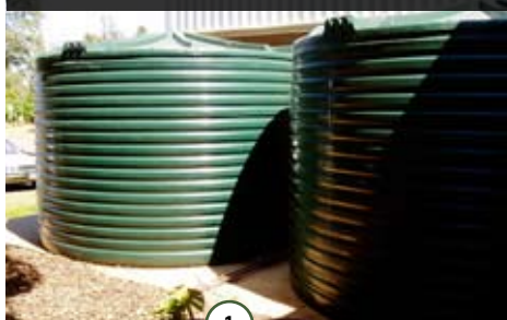
NEW TANK SYSTEM OUTSIDE O3 BLOCK
